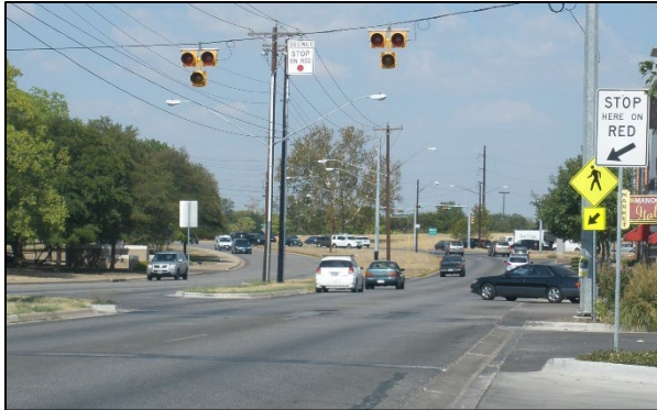
Pedestrian hybrid beacon – no stop required if no signal is displayed.
