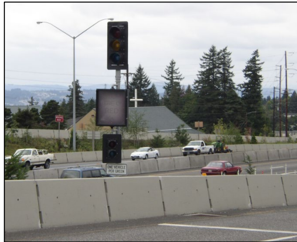
Freeway entrance ramp control signal – no stop required if no signal is displayed.
