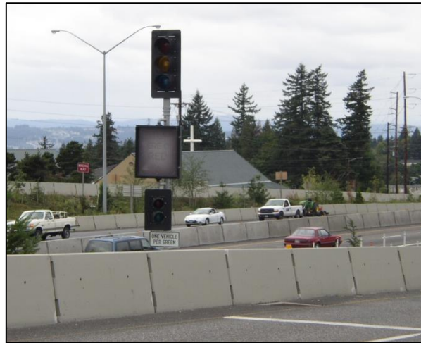
Freeway entrance ramp control signal – no stop required if no signal is displayed.
