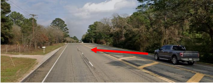
Crossing Prohibited (flush median)
